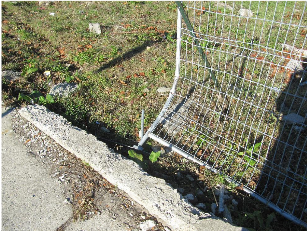
Figure 14: View of the deformed vertical post of the fence at the east end of the hole.
