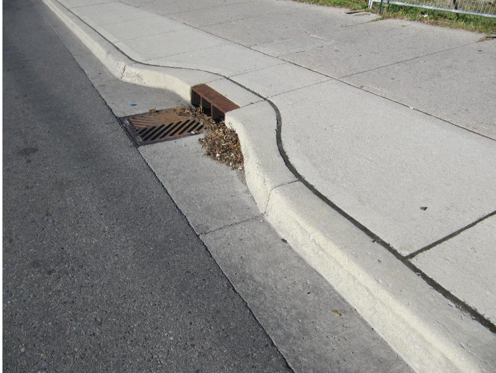
Figure 8: View of the sewer drain. A tire marks can be seen on curb just east of the drain and a close-up of that mark is shown in Figure 9. This mark would have been caused by one of the right side tires of the SUV.
